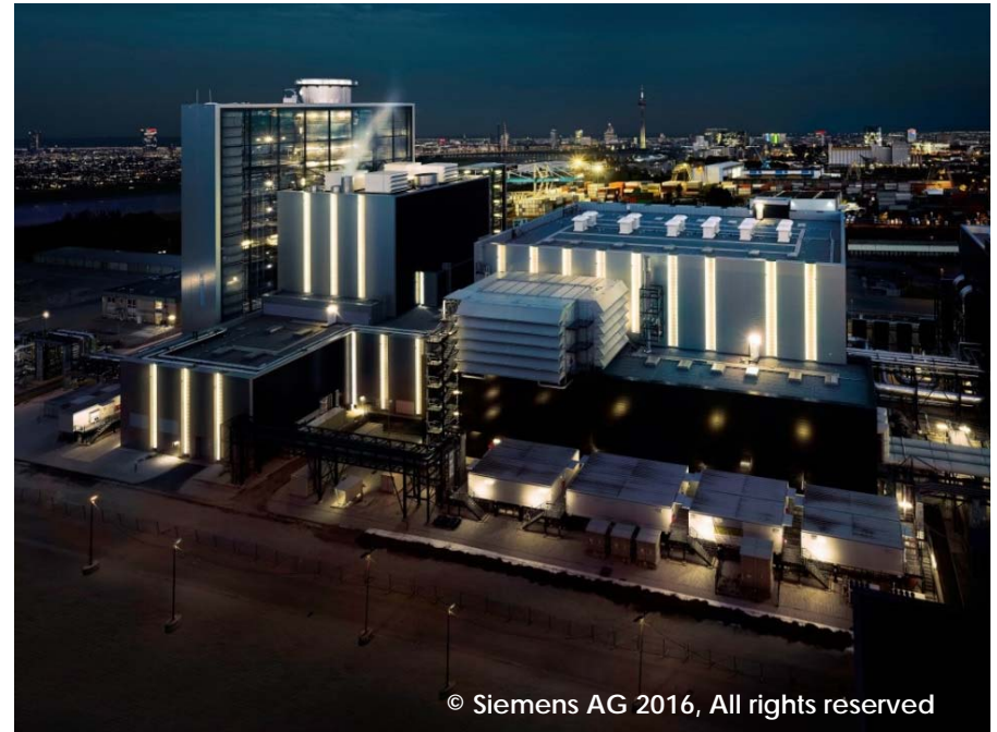
Lausward combined cycle power plant, Düsseldorf Germany
